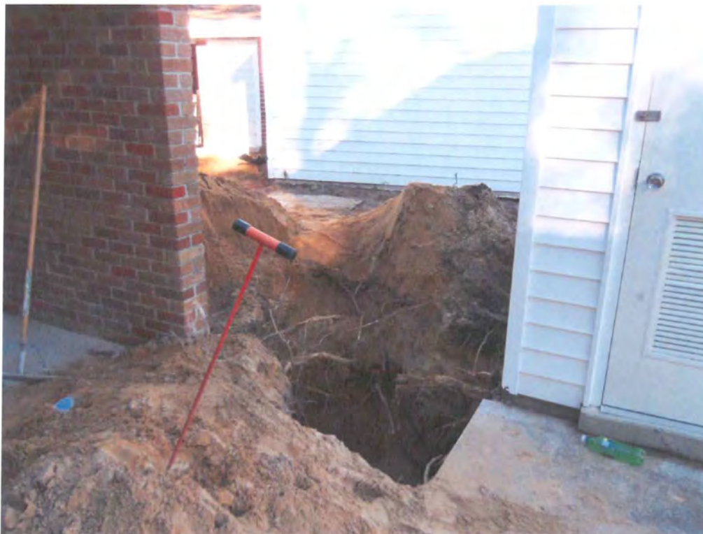
Picture 2: UST 586Aster excavation.
